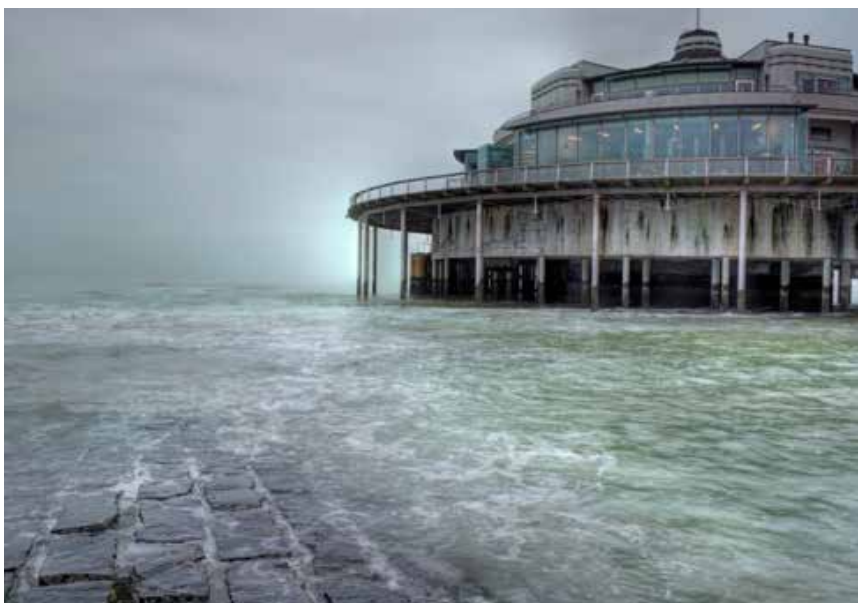
©Carl De Keyzer, Moments before the flood – Blankenberge Belgium - 2006
